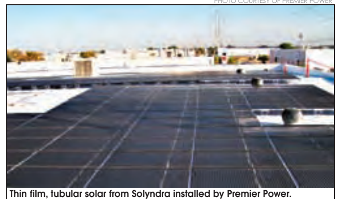
Thin film, tubular solar from Solyndra installed by Premier Power.
