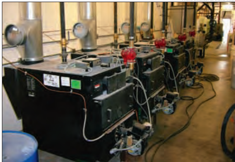
Waste oil boilers heat water for in-floor radiant heat, ice melt and hot water for a carwash. Used oil is becoming more attractive as the prices of conventional fuels rise.
