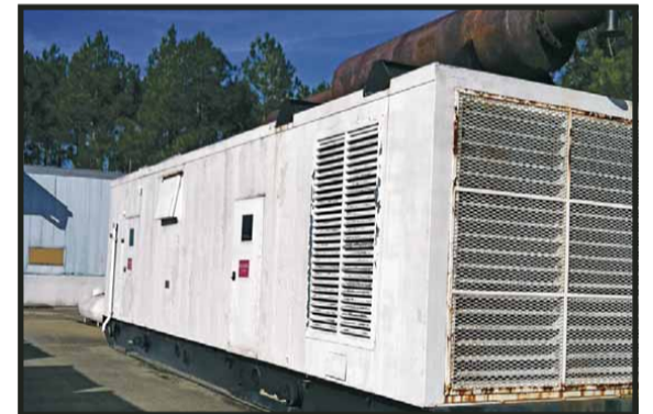
SELF-CONTAINED 750KW GENERATOR
