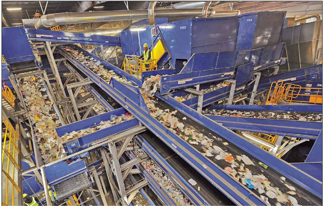
MSW System Running: Highly automated optical sorting systems are at the heart of advanced mixed material recovery facilities.
