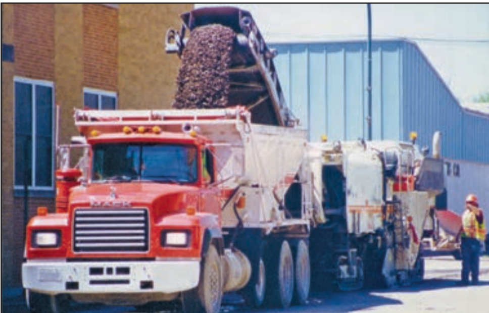
Old asphalt is milled off of roads, and immediately recycled on-site into material for the replacement roadway. The challenge is convincing states to allow mixes with a higher percentage of recycled content.
