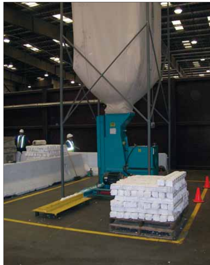
Equipment such as this densifier is necessary to compress expanded styrene packaging to prepare materials for recycling.
