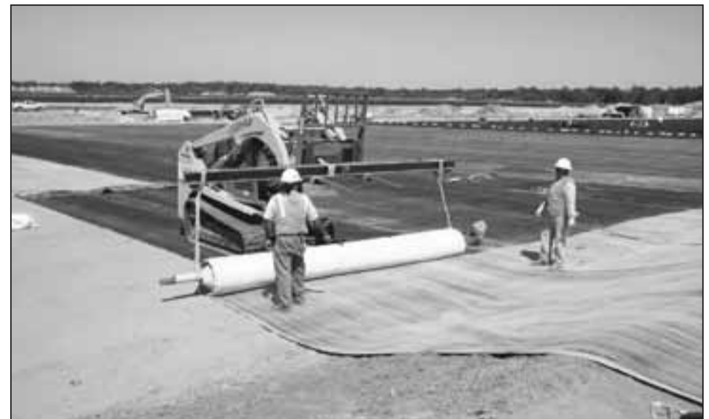
The plastic liner is considered the primary containment system. Should that rupture, however, any leachate would still have to penetrate the hard clay liner beneath it, meaning that contamination risks are slight.
