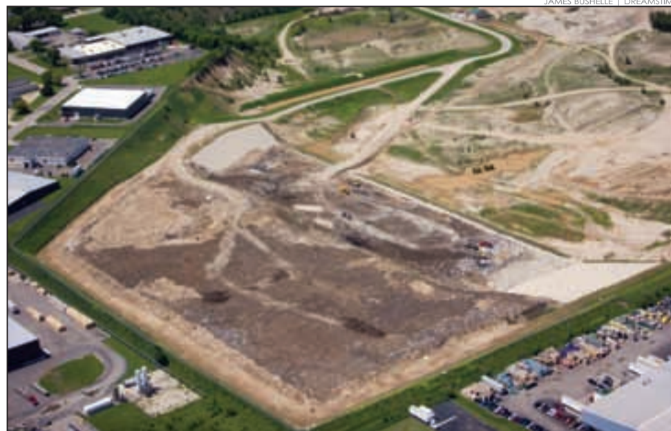
Generation equipment can be scaled down to small landfills, or modularly scaled up with additional engines or turbines as landfill gas flows increase.
