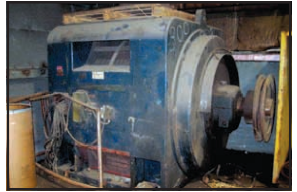
FAIRBANKS SHREDDER MOTOR
