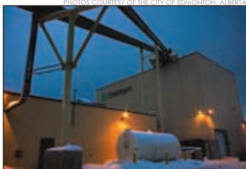
PHOTOS COURTESY OF THE CITY OF EDMONTON, ALBERTA Enerkem's first commercial plant in Westbury, Quebec transforms used utility poles into ethanol. The two conveyers connected to the roof take the shredded wood waste from a sawmill in front of the plant into the chemical process.
