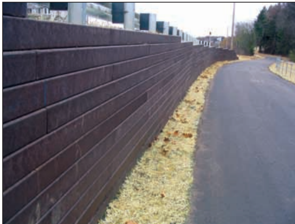
This large retaining wall in St. Paul, Minnesota utilizes recycled plastic lumber. It has the color and texture of railroad ties, but has the strength and durability of plastic.
