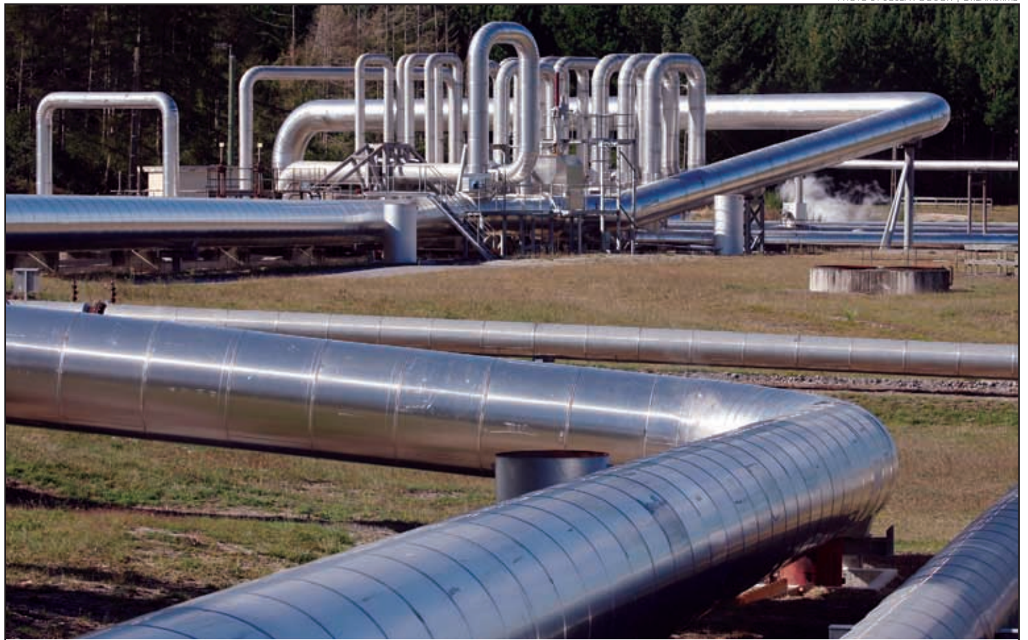
Insulated pipework at a New Zealand geothermal energy facility helps tap the unlimited supplies of energy generated by the earth's heat. While geothermal energy is clean and virtually limitless, economic considerations have prevented it from becoming as popular as solar or wind power.
