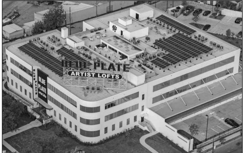
The Blue Plate building, an entry in the National Register of Historic Places, is one of the housing projects included in a Louisiana historic redevelopment project that will utilize Mage Solar products.
