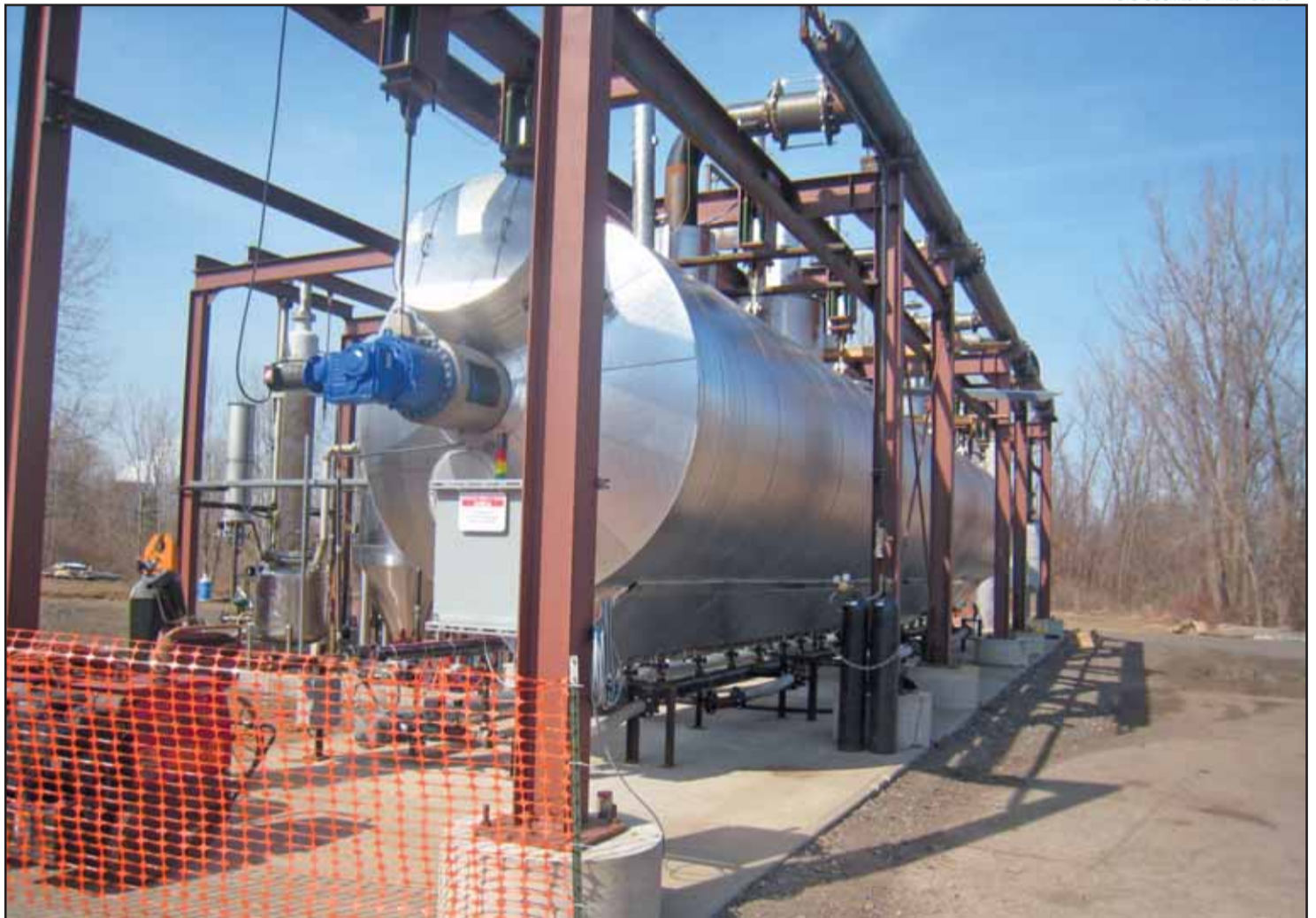
RES Polyflow's recently completed pyrolysis facility can turn approximately 10 lbs. of waste materials into one gallon of oil.
