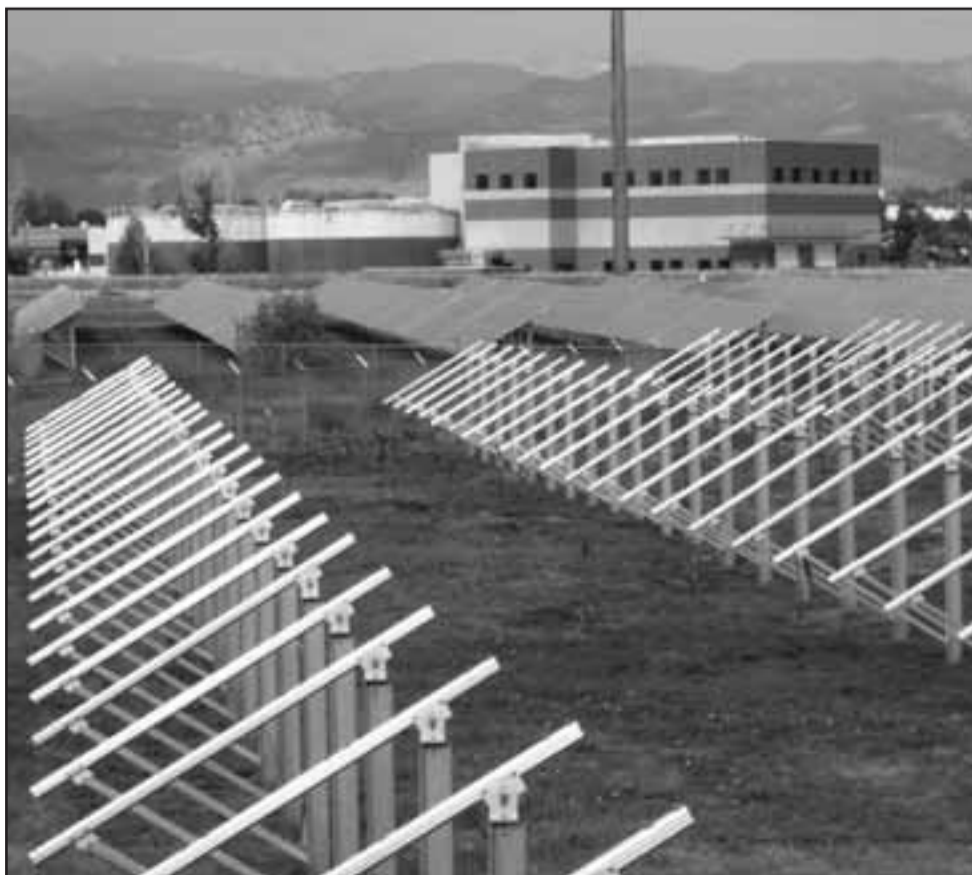
The City of Boulder, Colorado is nearing completion of a one megawatt solar electric system that will help power its wastewater treatment plant.
