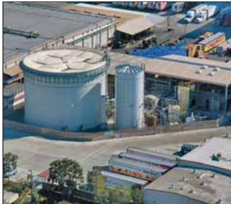
The innovative solution to convert food waste to clean energy was implemented at Kroger's Compton, California facility.
