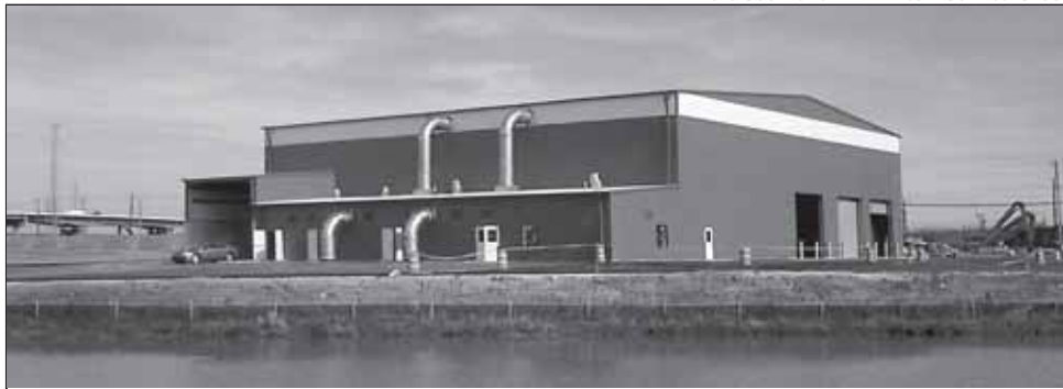
The Peninsula Compost Group's Wilmington Organic Recycling Center sits on 27 acres across from the Port of Wilmington, Delaware. The location was formerly a brownfield site that was remediated prior to construction.
