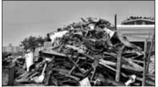
Waste Management's new sorting line can process up to 35 tons of C&D material per hour.
