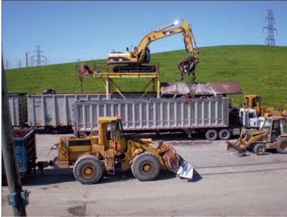
Republic uses a stanchion-mounted excavator to unload gondola railcars at Niagara Falls Landfill in Buffalo, New York.
