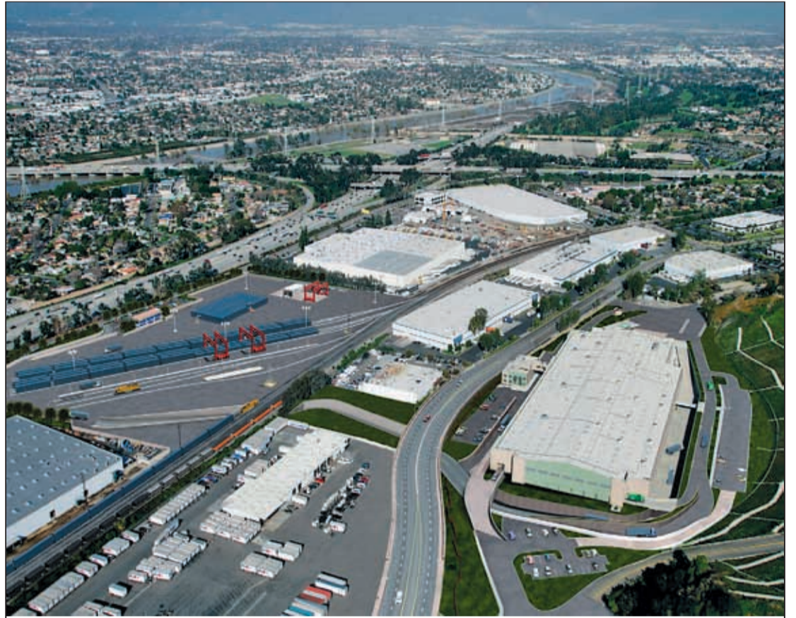
Artist rendering of rail yard currently under construction by Los Angeles County Sanitation Districts. Puente Hills MRF (far right) has a dedicated access road to bring loaded waste containers to a rail yard and retrieve empties.
