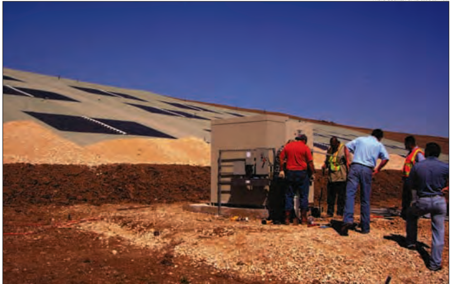
Workers install the inverter unit that converts solar DC current into AC. The white strips dividing the black solar panels are wire chases that carry DC from the thin film panels to the inverter for conversion.
