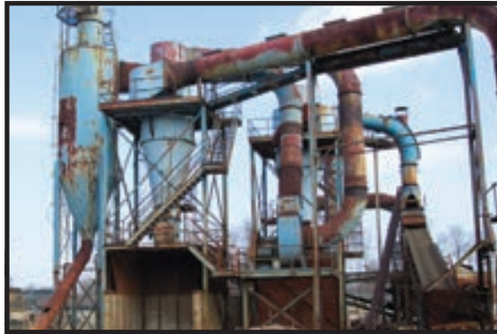
1994 MET PRO 74 x 104 AUTO SHREDDER Complete 4,000 h.p. ferrous shredding system. $1,450,000
