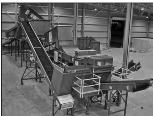
—A completed Remcon installation in Sweden
