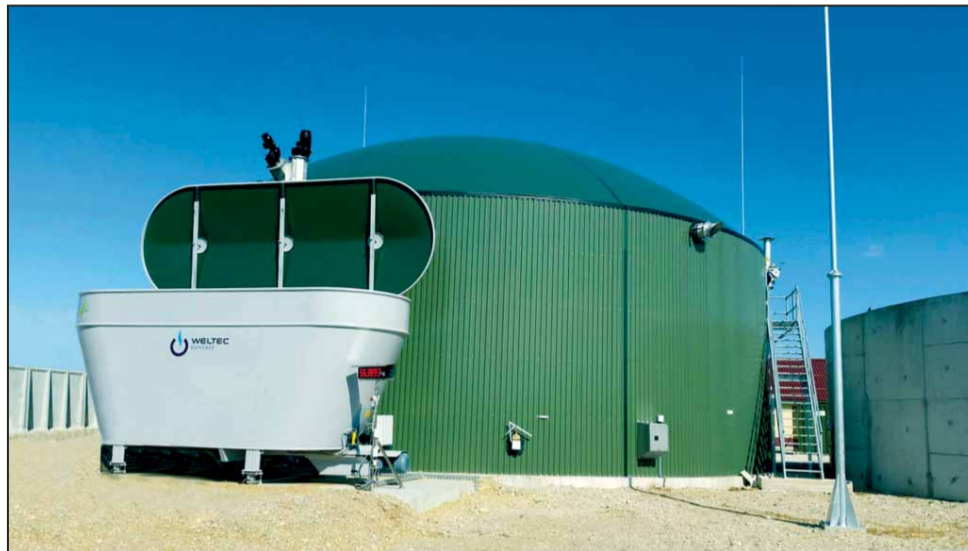
In view of the liquid manure share, a small 35-m 3 input system is sufficient for transferring the solid substances, such as maize silage.
