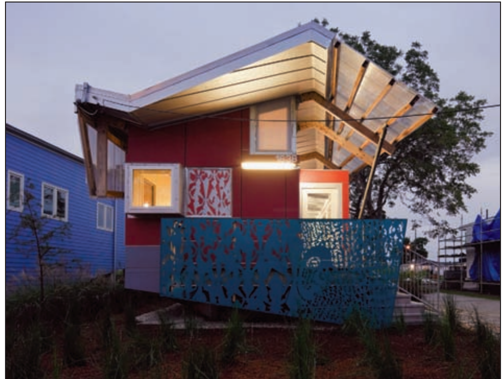
In the event of flooding, the base of the house acts as a raft and allows the house to rise vertically on guide posts – up to twelve feet – as water levels rise.
