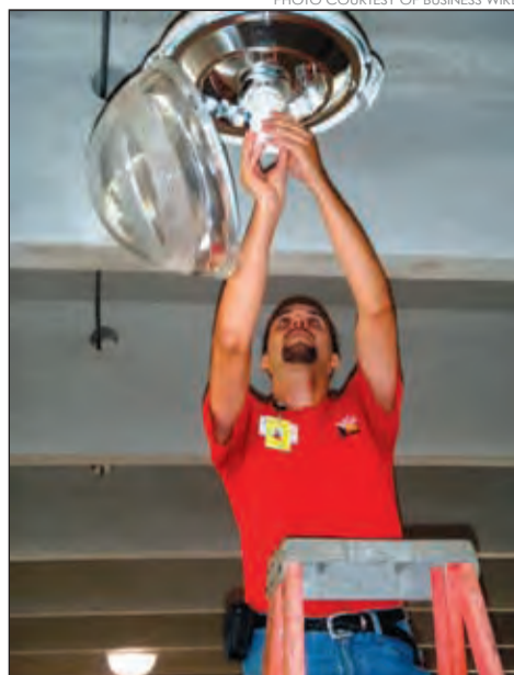
An Office Depot associate changes out a garage light from a 130 watt metal halide lamp with ballast to a 54 watt fluorescent light.
