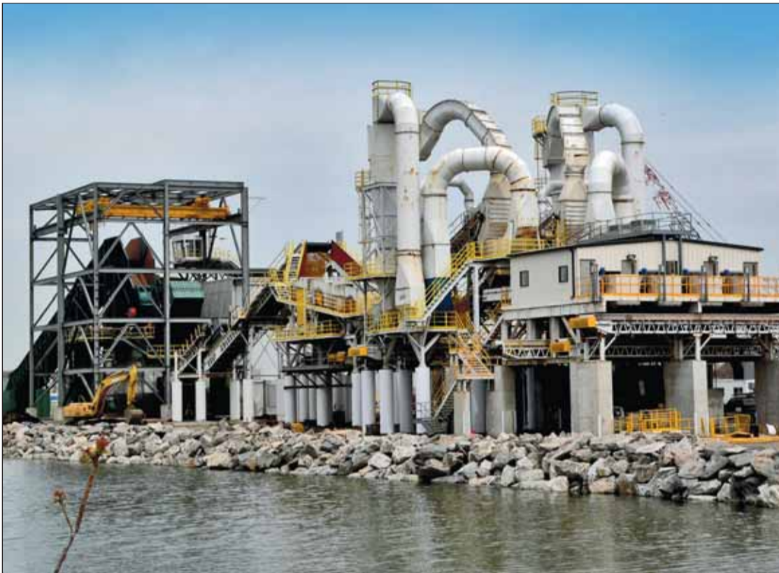
Riverside Engineering's MegaShredder in Jersey City, New Jersey is a 122" in diameter, 112" wide, powered with a 9,000 hp main drive motor with a capacity of 350 tons per hour.
