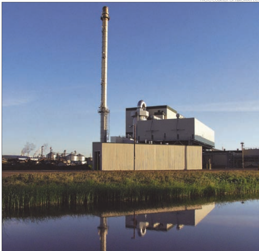
The Fibrominn plant in Benson, Minnesota generates electricity by combusting turkey litter and biomass and provides an outlet for growers to dispose of excess litter and earn income.
