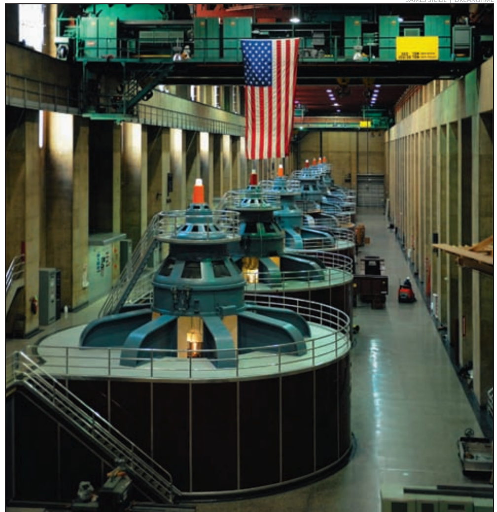
Although large hydroelectric operations like this one have potential to generate quite a bit of green energy, some believe that even more energy could be harnessed by a large number of smaller facilities.
