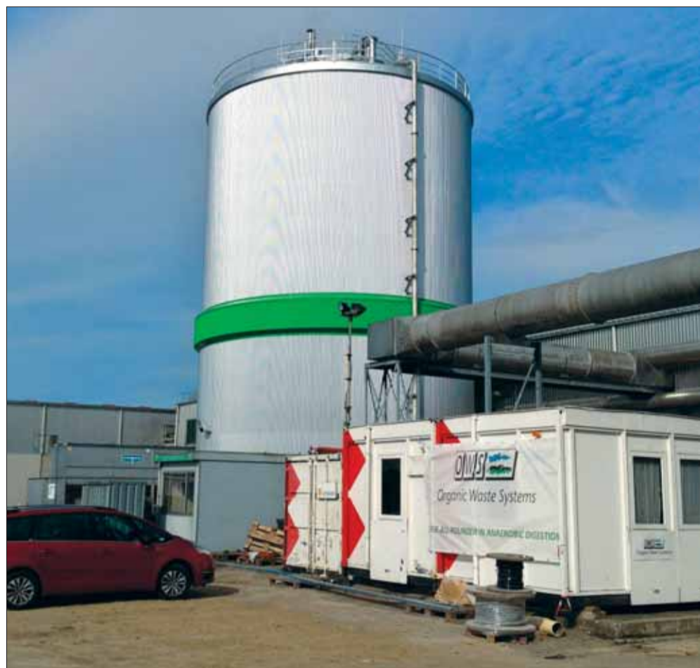
Organic Waste Systems' second plant in Wijster, Netherlands. It processes 44,000 tons per year of biowaste, including food waste, yard waste, soiled papers and compostable packaging. Plant started up in May 2013, the second OWS digester at the site owned by Affero BV.
