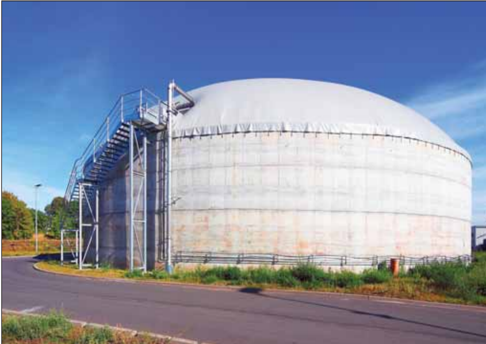
Anaerobic digestion plant at Michigan State University. Manure, food waste and other organic matter go into the airtight tank, which holds about 450,000 gallons. Contents are maintained at roughly 100 degrees Fahrenheit for 20 to 30 days. The result is biogas and a slurry of partially decomposed organic matter, water and nutrients.
