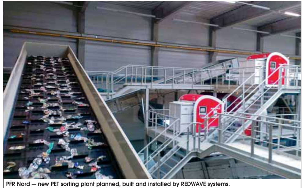
PFR Nord — new PET sorting plant planned, built and installed by REDWAVE systems.
