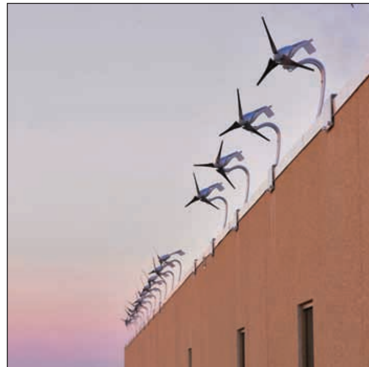
Roof-mounted wind turbines provide electrical power at Kettle Foods' Oregon facility.
