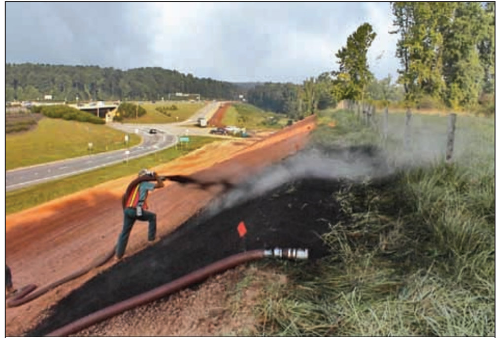
A worker completes compost application beside a highway.
