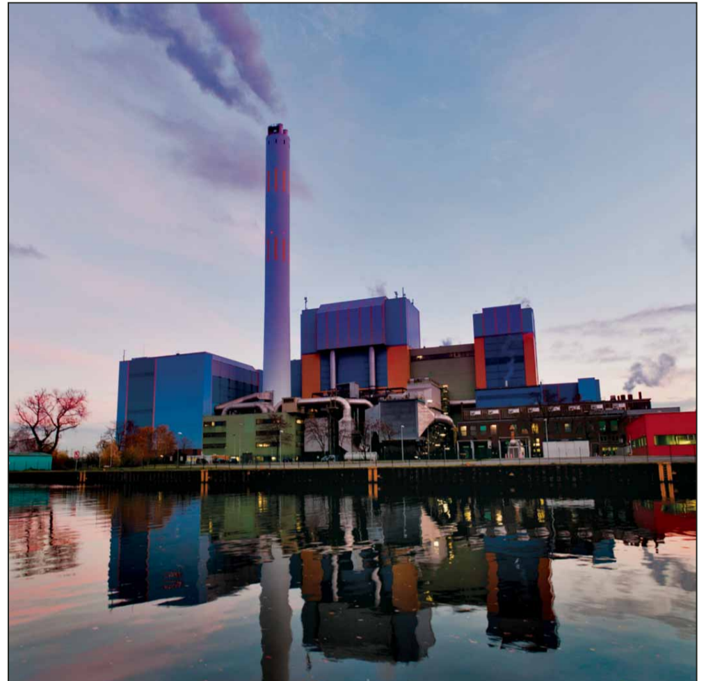
Building complex of a modern waste-to-energy facility in Oberhausen, Germany where a higher concentration of facilities is seen in space restricted countries.
