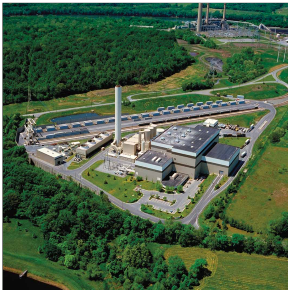
Covanta's Montgomery County facility.
