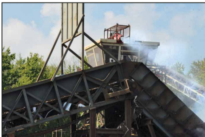
Buffalo Turbine LLC
