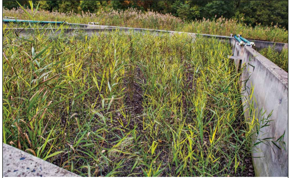
RMC recognized the use of recycled glass as a growing medium for the reed bed filtration system at the Authority's Beam road wastewater treatment plant.
