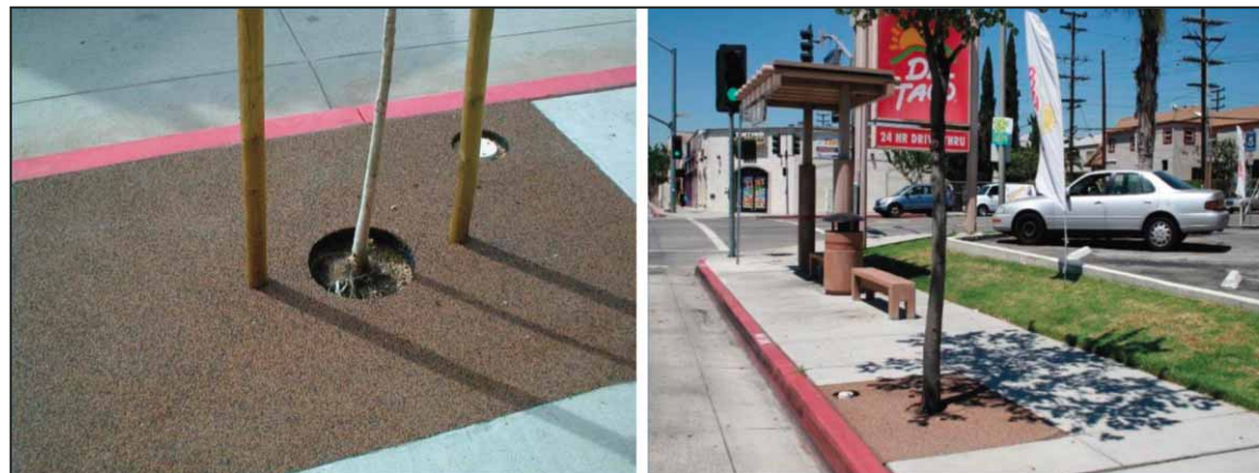
The City of Glendale, California uses tree wells made by United Sports Surfacing of America from recycled tire rubber. They are low cost and avoid metal grates that cut into growing trunks. The tree wells allow the surface to be cut to accommodate tree expansion.
