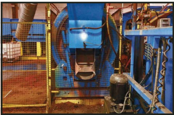
RUBBER MULCH PAINT LINE
