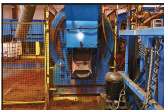
RUBBER MULCH PAINT LINE
