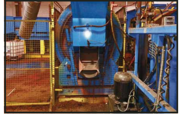
RUBBER MULCH PAINT LINE
