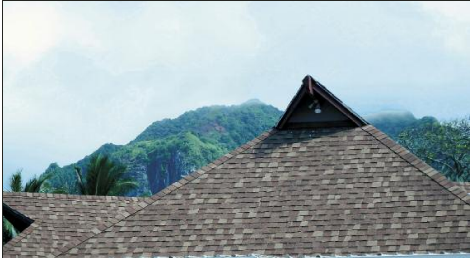
Rubber roofing tiles are one of the many tire-derived products available on the market today.
