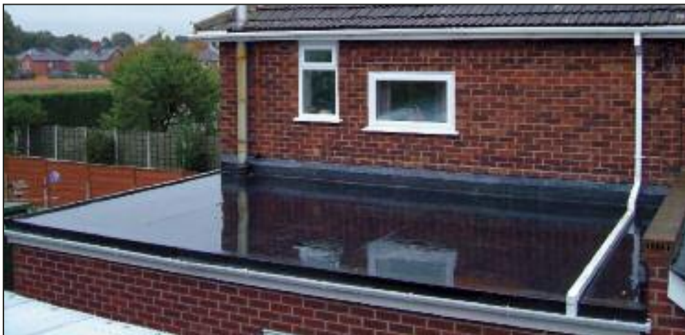
Rubber membranes for flat roofs or for those with a slight slope are usually manufactured from EPDM rubber. EPDM refers to the following rubber types: ethylene, propylene, diene and the M refers to it's classification.
