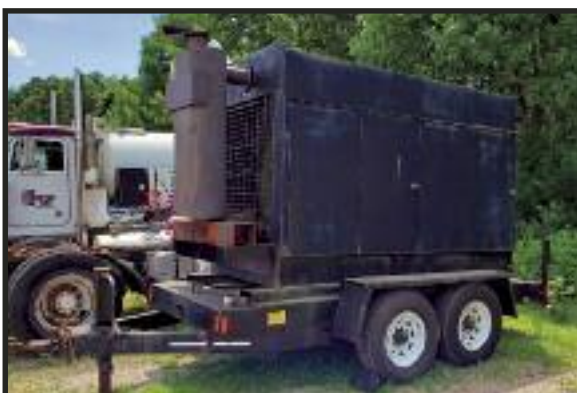
LEROY SOMER PORTABLE 250KW GENERATOR
