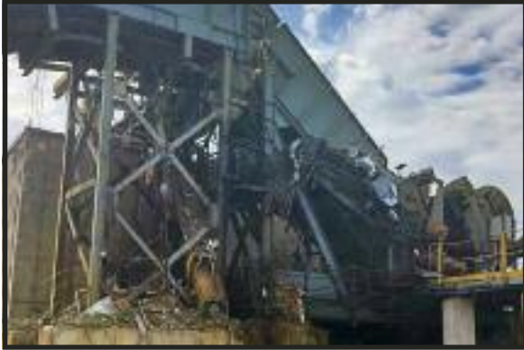
2012 HARRIS 60 x 90 HAMMERMILL SHREDDER 2000HP complete ferrous shredding operation!
