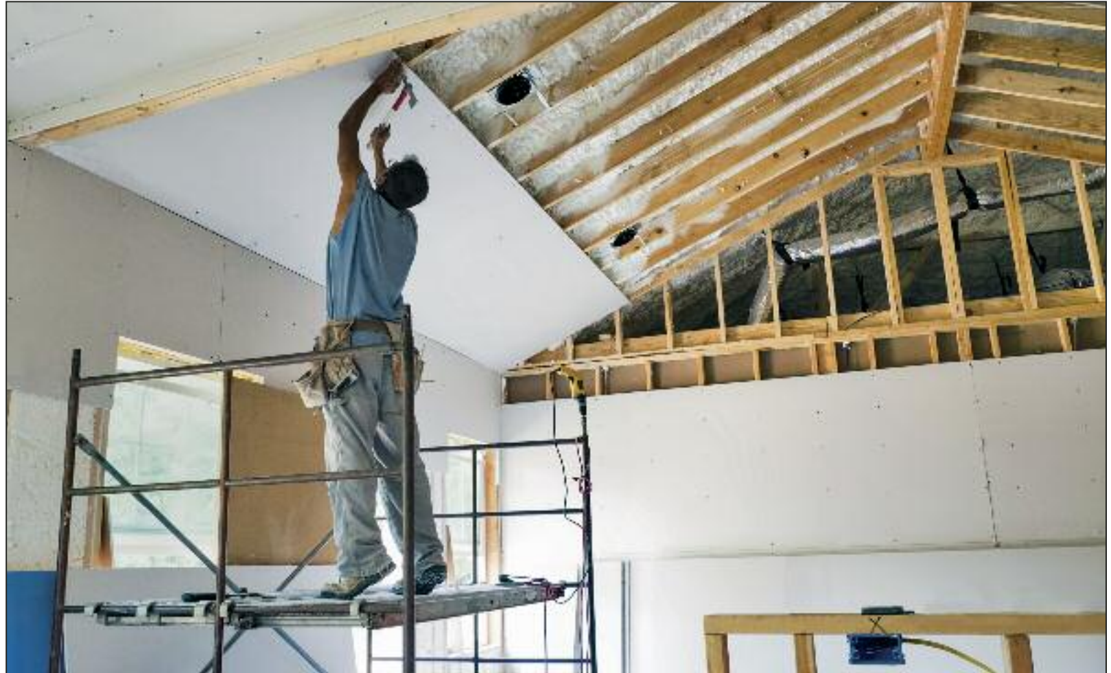
Gypsum is widely mined and is used as a fertilizer and as the main constituent in many forms of plaster, blackboard chalk and drywall. Gypsum board is commonly known as sheetrock or plasterboard.
