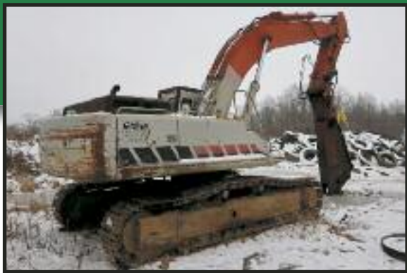
LINK BELT EXCAVATOR WITH LABOUNTY SHEAR
