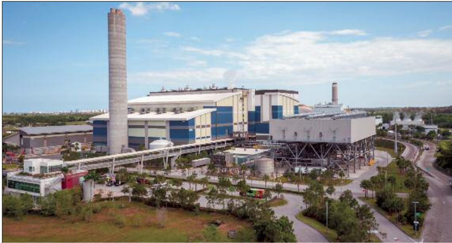
Covanta's waste-to-energy facilities are designed to convert remaining waste after recycling by combusting it – generating steam for electricity production. Leftover ash is then processed to recover metal for recycling while all gases are collected, filtered and cleaned to minimize environmental impact. PHOTO COURTESY OF COVANTA
