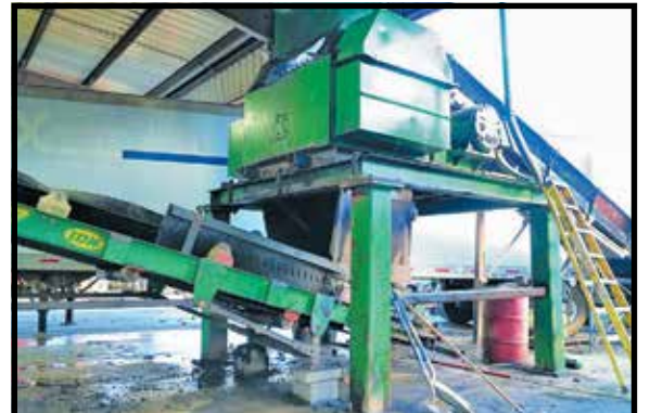
CM MULTISTACK TIRE SHREDDER SYSTEM ROTOR RECENTLY REBUILT! INCLUDES CONVEYANCE.
