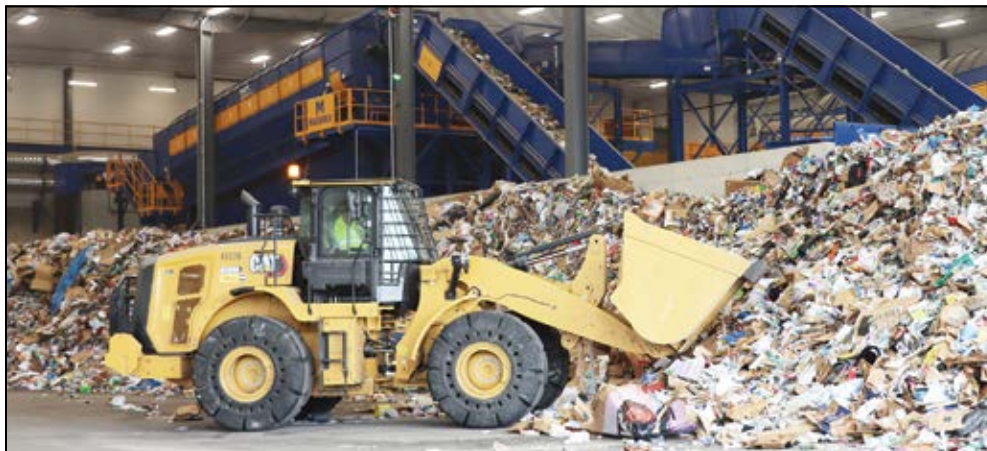
Material is dumped from the collection trucks to the tipping floor. The new Rumpke facility processes materials from 50 different Ohio counties and has the capability to process 250,000 tons annually. A separate tipping floor exists for commercial loads.
